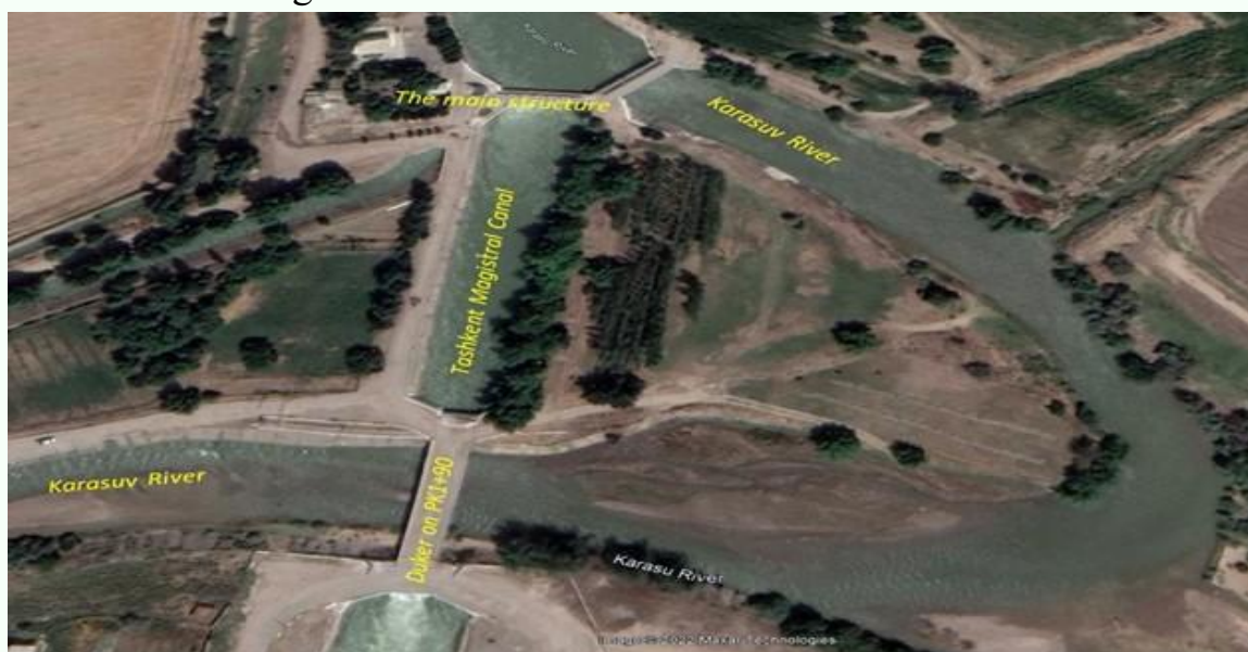
Figure 3. Satellite view of the head section of the Tashkent Main Canal.
